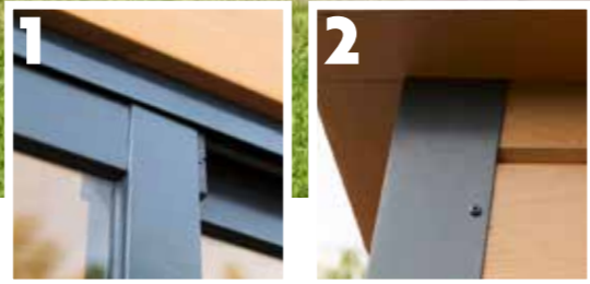
1. Sliding door with aluminium frame 2. Edge protector in aluminium
