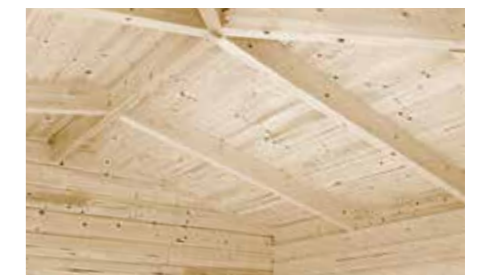
18 mm roof boards
